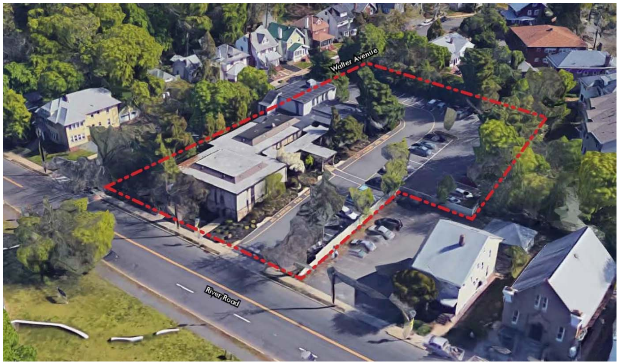
Figure 2: Bird's eye view of Redevelopment Area
