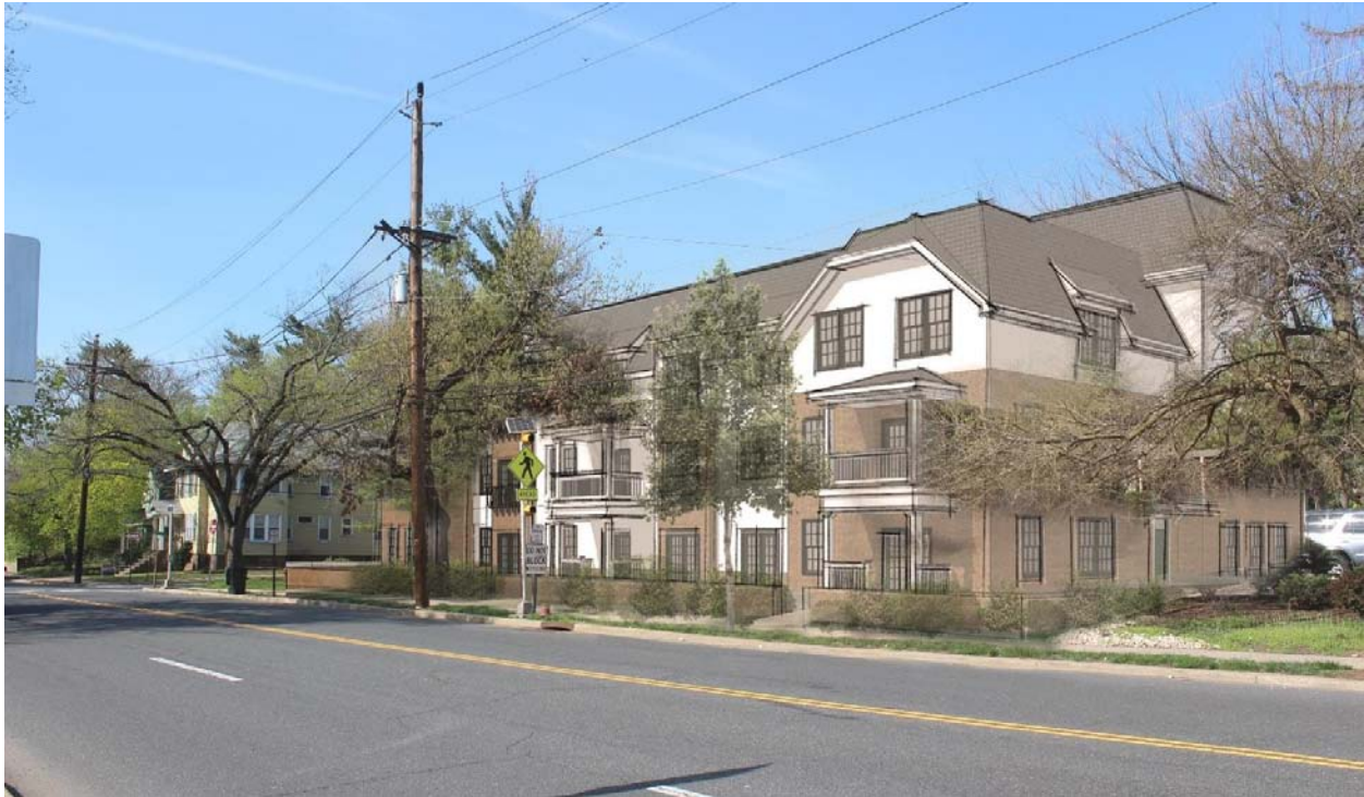
Figure 15: Rendering of potential massing and character in accordance with the Redevelopment Plan as viewed from River Road; note the use of low-walled terraces and balconies to enhance livability along a busy road and take advantage of river views
