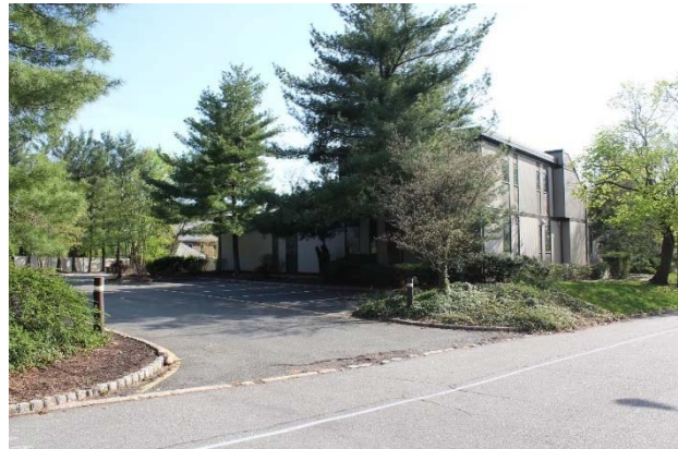
Figure 4: Street view of Redevelopment Area from Walter Avenue
