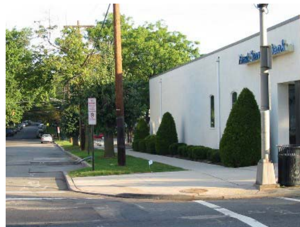
Several streets in Highland Park have curb extensions. This curb extension on North Third Avenue at Raritan Avenue is only four feet wide; more effective extensions would be six to eight feet in width.
