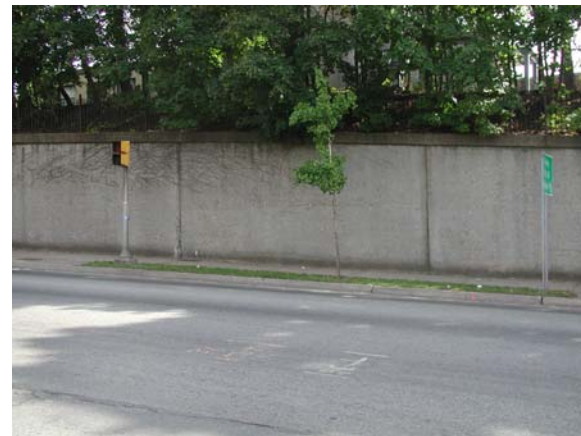
Retaining wall at Raritan Gateway
