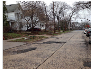
Concrete Road Segment
