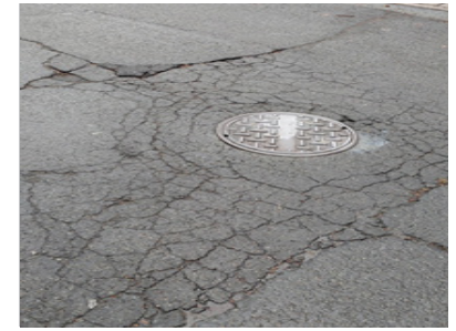
Alligator Cracking
