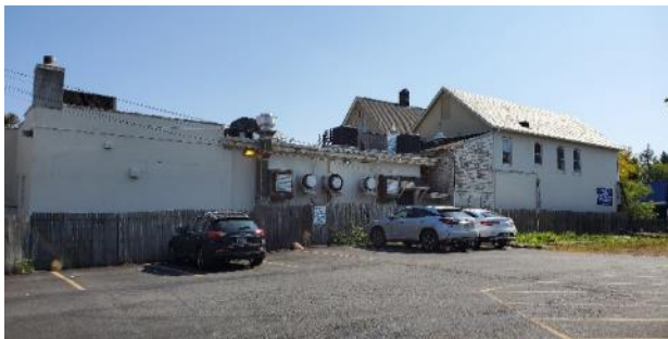
View of west side of existing building on Block 1603 [162]
