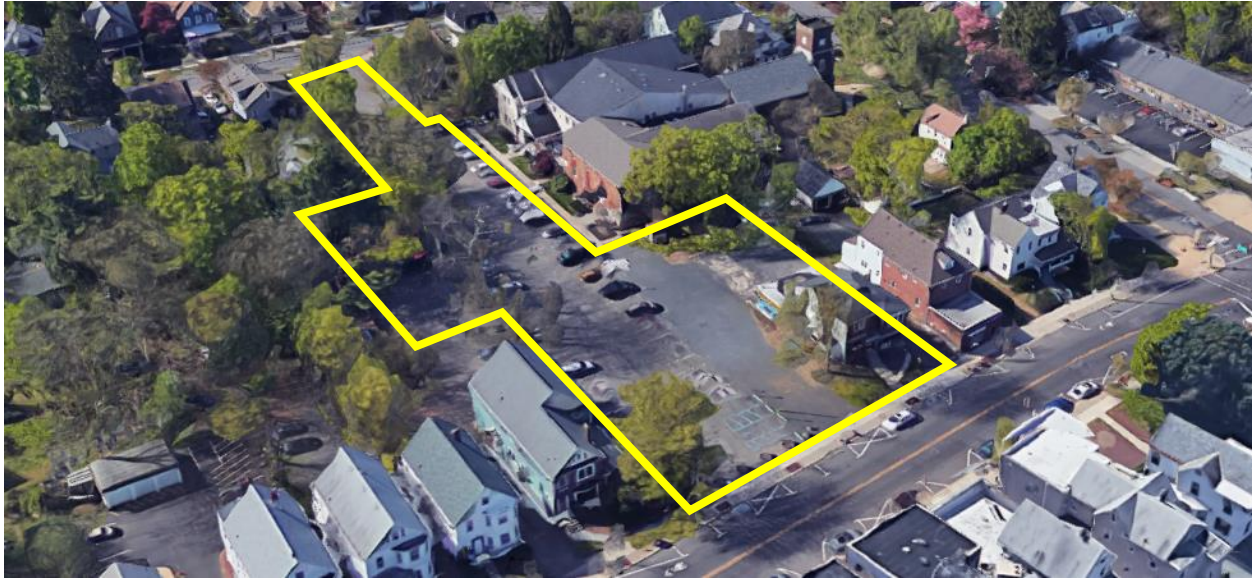
Google Maps eye view of Tract C outlined in yellow, looking southwest.
