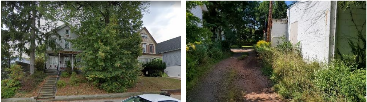
Google Maps Street View of Tract B from Raritan Avenue. View of alley along rear of Tract B.
