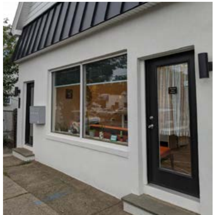
106 Woodbridge Avenue: After
