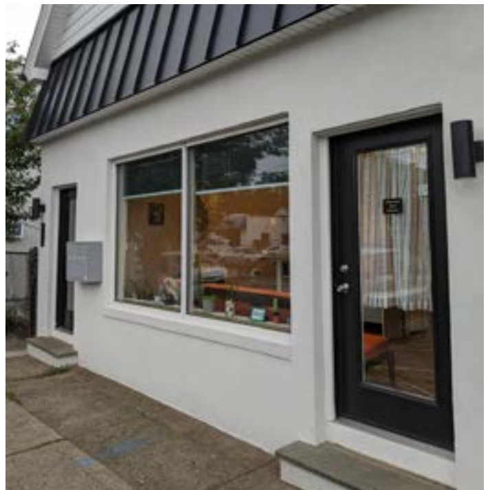
106 Woodbridge Avenue: After
