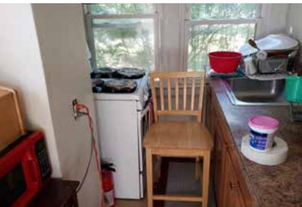
At least one outlet was exposed without its protective cover and at least one extension cord was being used to power other devices.
