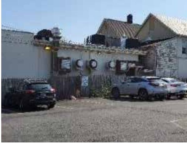
View of west side of existing building on Block 1603.
