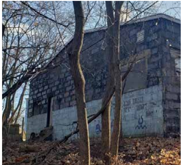
View of building at rear of Tract A.
