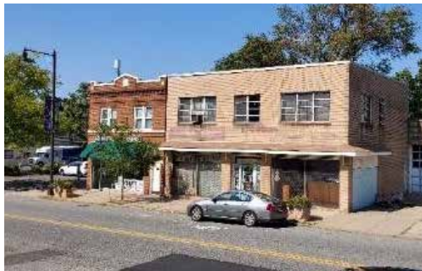
View of Classic Cleaners and former Gun & Boat buildings from Raritan Avenue.
